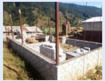
[Reinforced Masonry Structural Wall System] Those buildings which falls under this typology shall be inspected using
