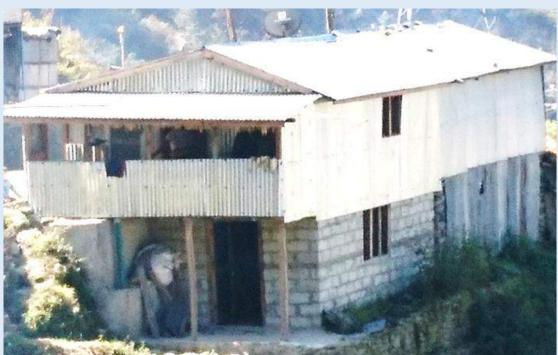
Hybrid Structure [Upper Storey : Light Timber Frame Structure] [Lower Storey : HCB Structure]
