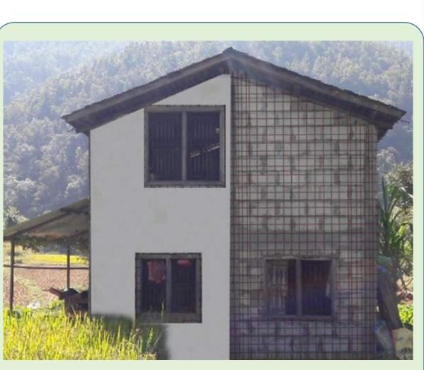
Figures : Jacketing of HCB building using GI wires and plaster
