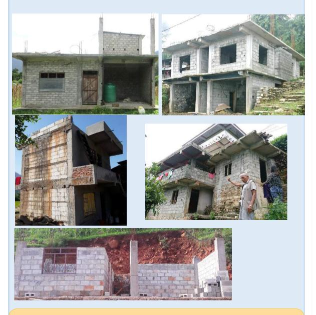
• [Exceptional Cases] : The rebar (in building infilled with HCB) can differ but shall be justify with Structural Analysis and Design.
