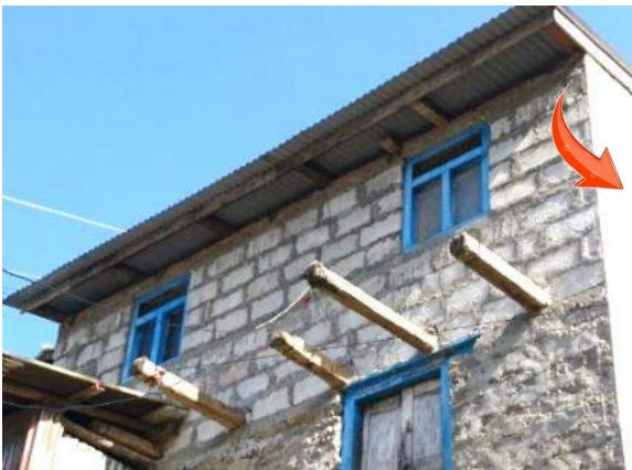
[If no practice columns are casted], Press the corner of the block in actual construction site where block edge is exposed or remove plaster (if required).
