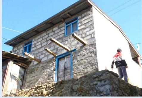
Hybrid Structure [Upper Storey : HCB Structure] [Lower Storey : Stone in Cement Structure]
